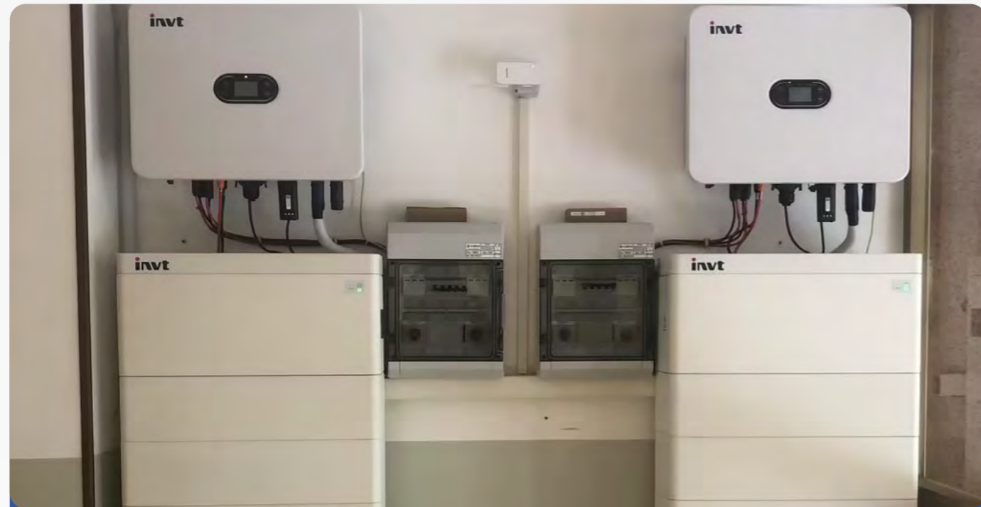
20kW+40kWh, Italy (XD10KTR*2, GRP2.56-S8HV*2)
