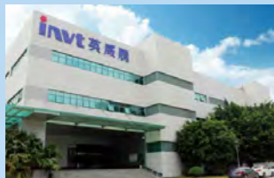
Shenzhen Fuyong Industrial Park
