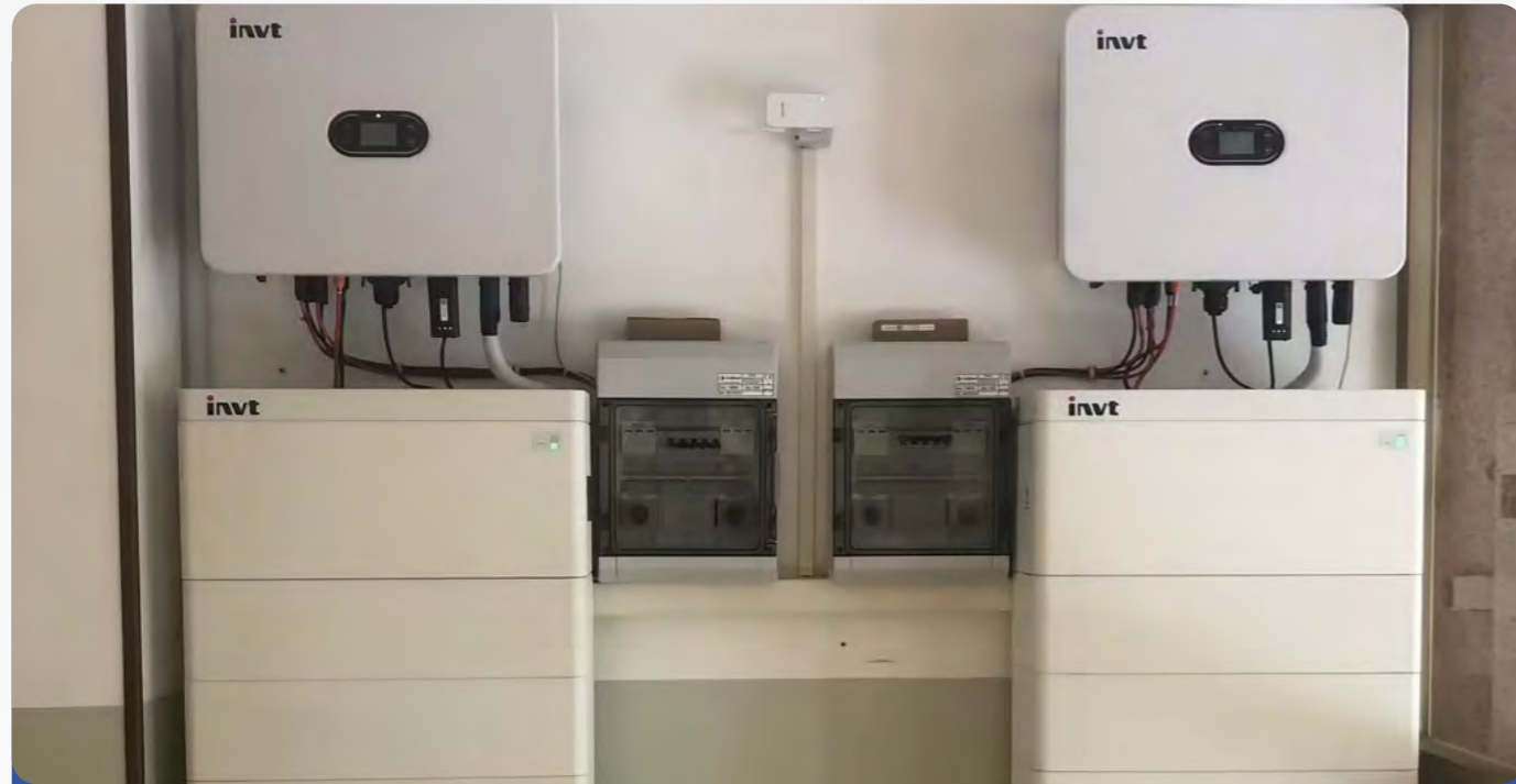
20kW+40kWh, Italy (XD10KTR*2, GRP2.56-S8HV*2)
