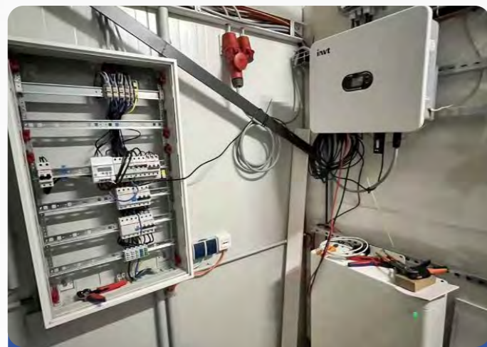
10kW+10kWh Germany (XD10KTR*1, GRP2.56-SHV*4)
