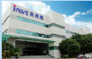
Shenzhen Fuyong Industrial Park
